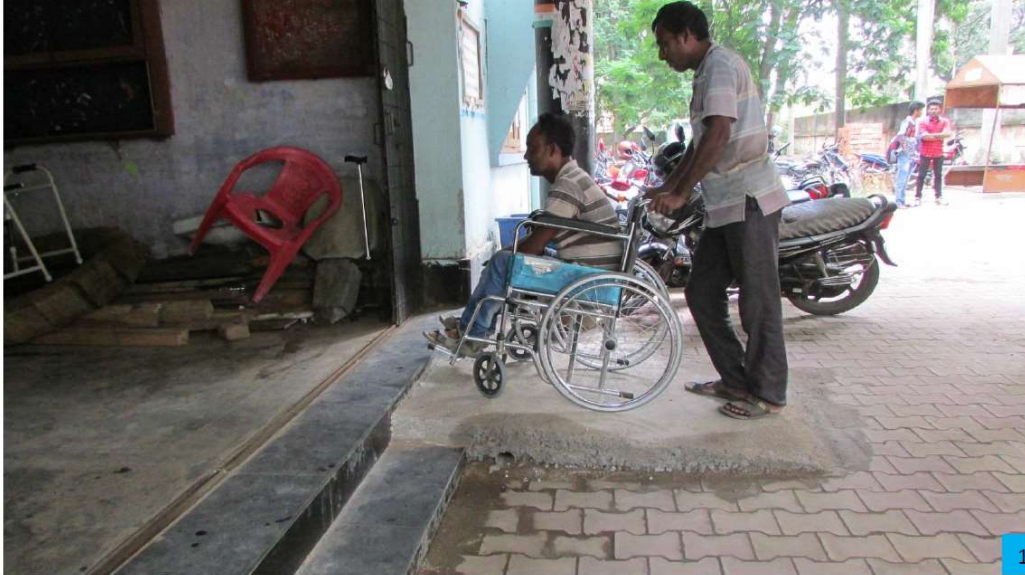
Figure 2: Ramp facility at Arts building
